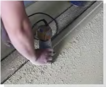
Step 3: Cover the corner needed, cut V style gap on the back side.
